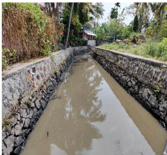
Storm Water Drainage at Thevara
