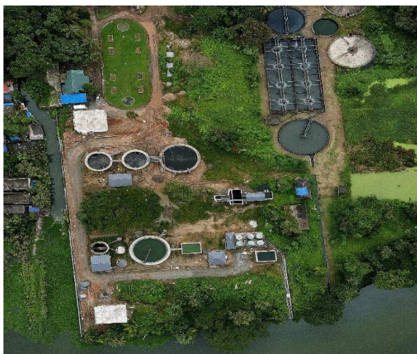
Sewerage Treat Plant (STP) at Elamkulam
