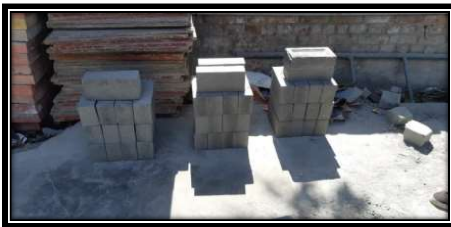
Figure 2: Casting at Akira marbles GIDC, New V U Nagar
