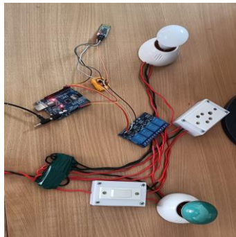
Fig.2 Smart Home Automation
