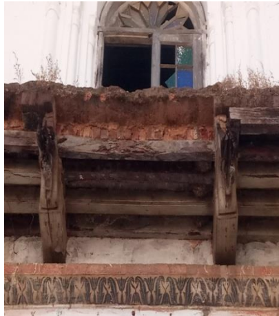
Fig 12- Slab edge deterioration due to mosses
