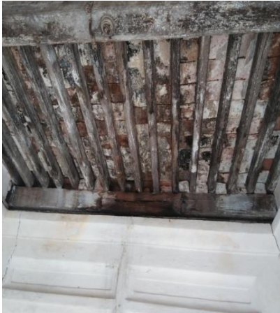
Fig 11- Damages in Roof plaster
