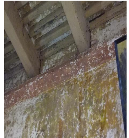
Fig 13- Cracks and joint failure
