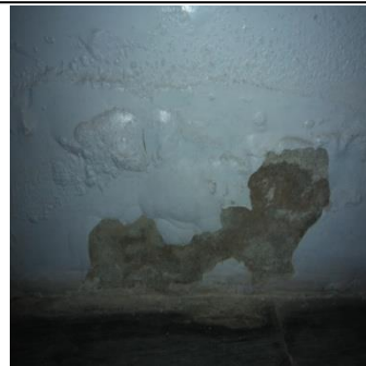
Fig 15- Spalling and moisture effect at Raghunath Palace
