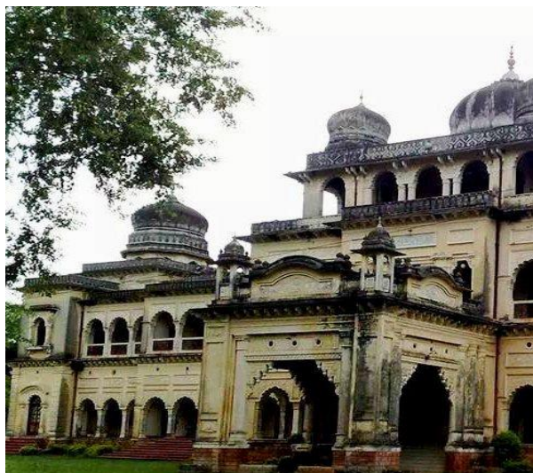
Fig 6- Kumar's Palace at Baikunthpur
